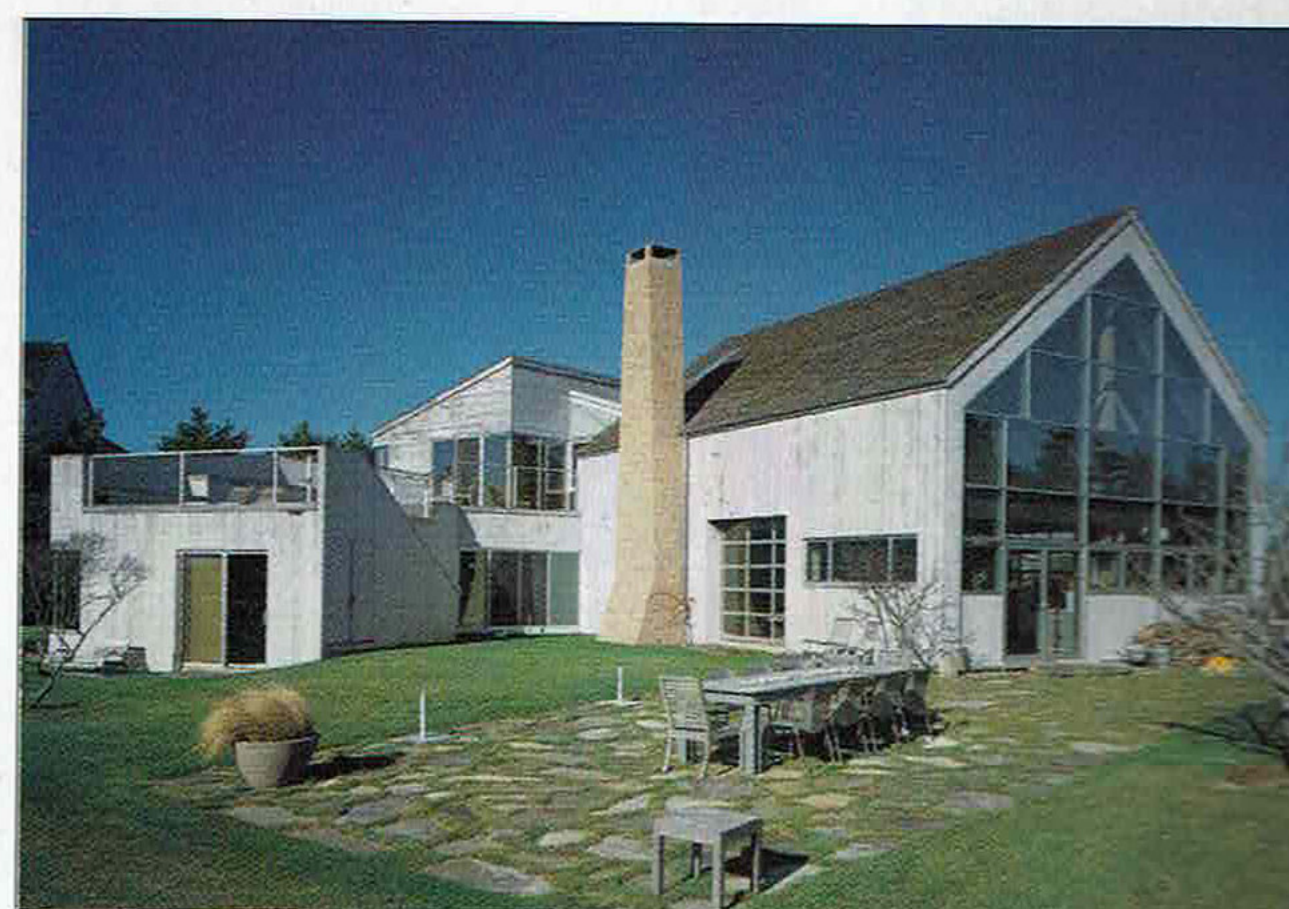
To celebrate a 220-year-old barn frame, architects Tom Hut and Jane Sachs built a 2x6 wood-frame house around the antique structure.
